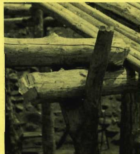
An older photo shows Douglas Fir poles that are stripped and then assembled to form the roof of the roundhouse.
